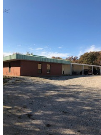
Brick office building (4,300 sq ft)
